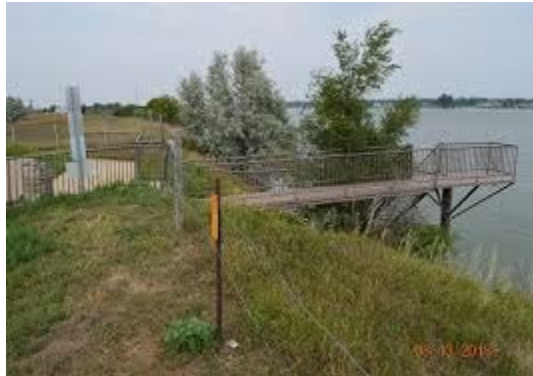
(Heskett Power Plant Stairway in 2018)
