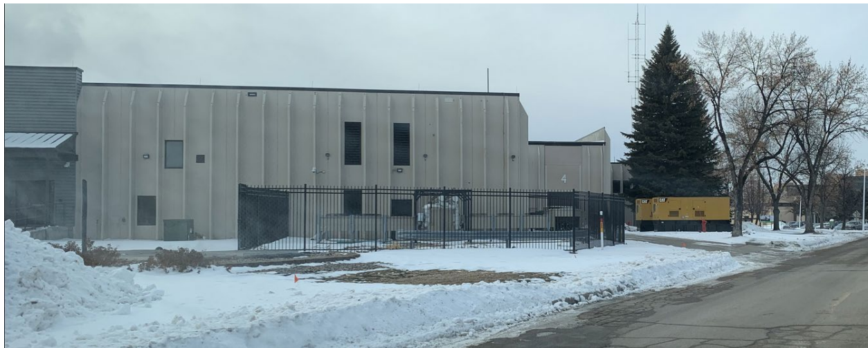
PHOTO SHOWING BOTH BACKUP GENERATORS AND HVAC EQUIPMENT (BEHIND FENCE). WHILE THE FENCE IS OF SUFFICIENT STRENGTH TO DETER VANDALS OR THIEVES FROM TAMPERING WITH THE EQUIPMENT, IT IS NOT STRONG ENOUGH TO PREVENT A VEHICLE FROM CRASHING THROUGH AND DAMAGING THE COOLING EQUIPMENT.
